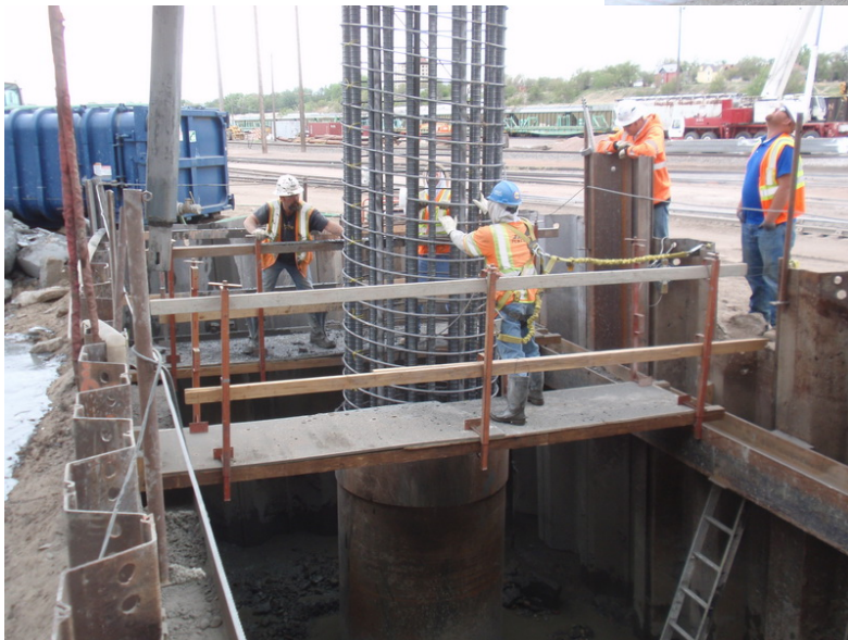
Figure 7 – EB Pier 5 Drilled Shaft Construction – May 13, 2010:
