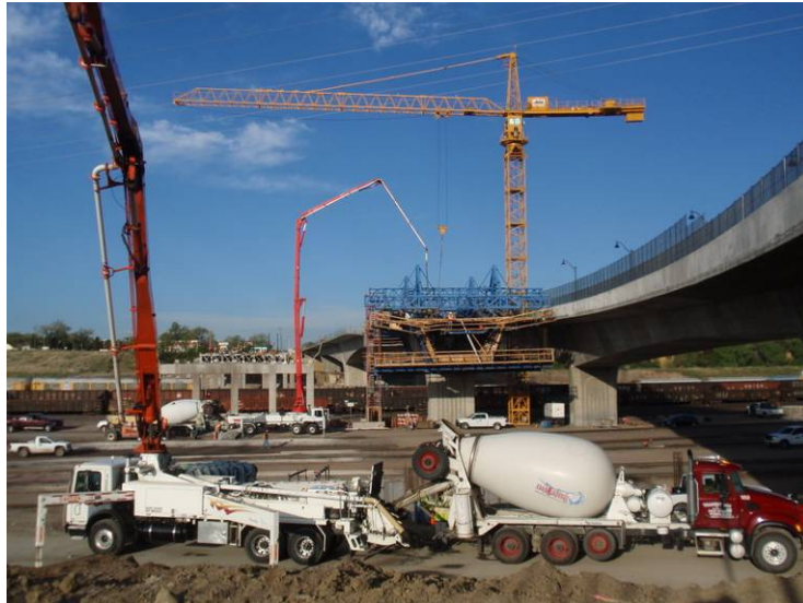
Figure 9 – EB Bridge Construction – May 21, 2010:
