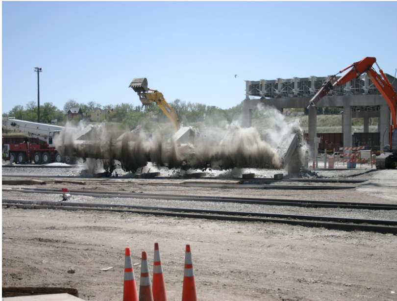
Figure 3 – Existing Bridge Demolition – May 10, 2010:
