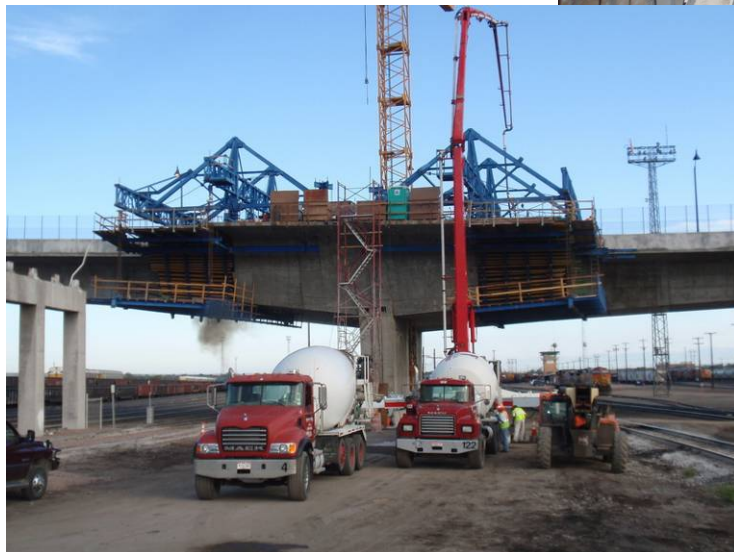
Figure 11 – Cantilever 4 EB Segmental Construction – May 21, 2010:
