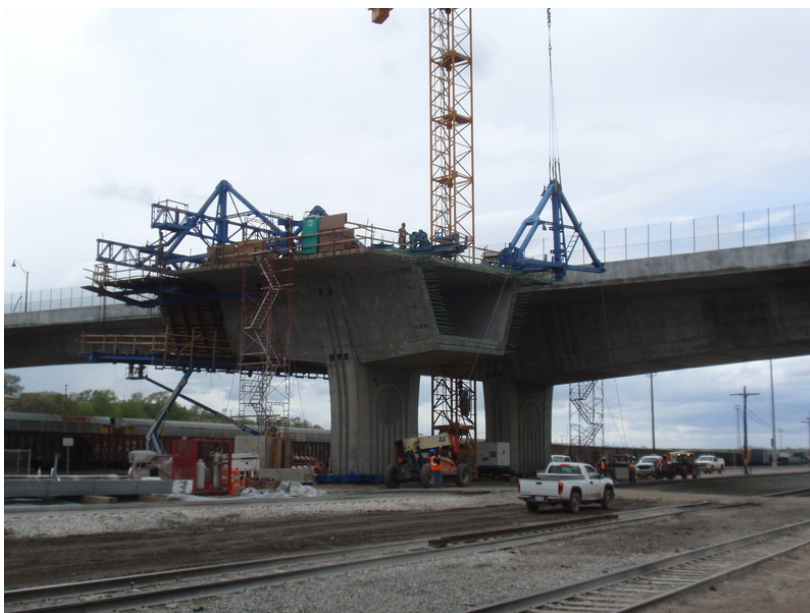
Figure 5 – Cantilever 4 EB Segmental Construction – May 12, 2010:
