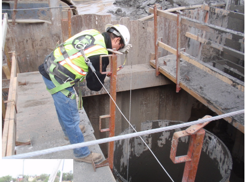
Figure 6 – EB Pier 5 Drilled Shaft Construction – May 13, 2010:
